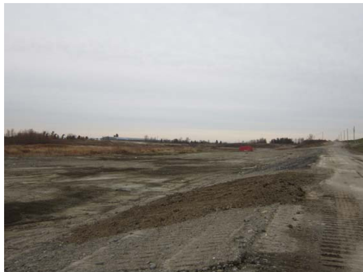
Image 4: Looking north at disturbances associated with grading and aggregate removal.
