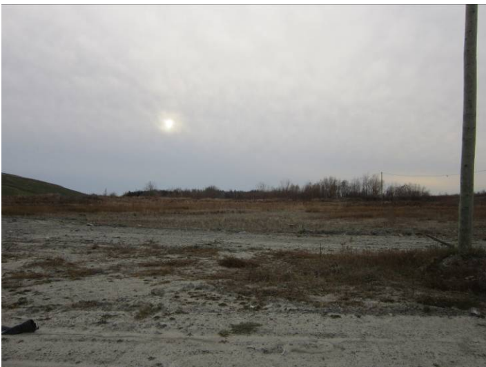
Image 3: Looking southeast at disturbances associated with grading and aggregate removal.
